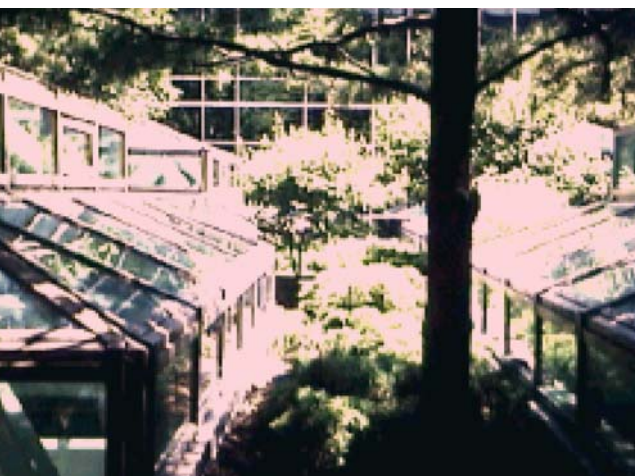
Fig. 4– Queen’s Quay Terminal Toronto, Ontario, Canada Green Roof Courtyard with Skylights Architect: Zeidler Roberts Photograph courtesy of M. Kuhn
