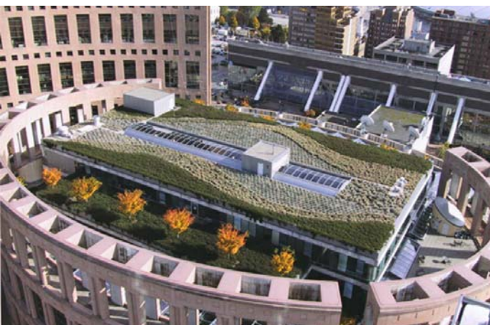
Fig. 12 – Vancouver Public Library Green Roof Vancouver, British Columbia, Canada Photograph courtesy of Hydrotech
