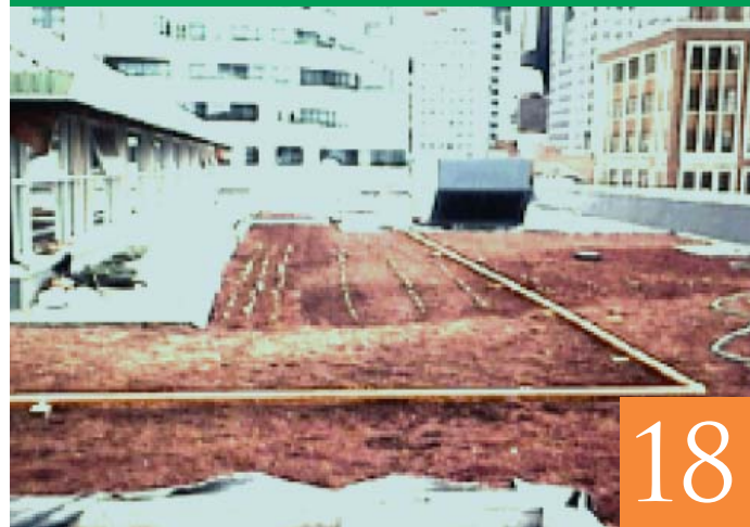
Fig. 11 – Mountain Equipment Co-op Toronto, Ontario, Canada Soprema Green Roof Installation and Planting Photograph courtesy of M. Kuhn
