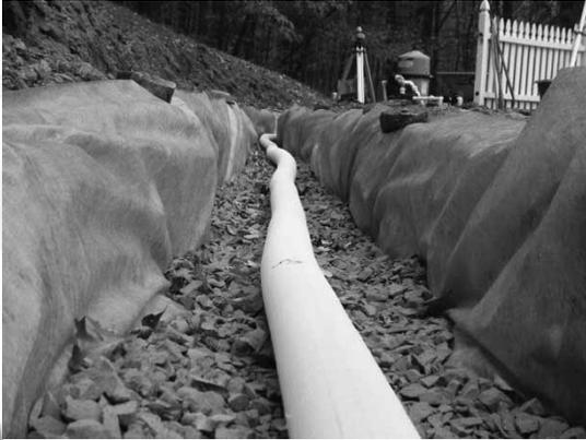
Soakage trenches can pollute groundwater if not properly sited, designed, and operated. They are regulated under the federal Underground Injection Control (UIC) program. Contact the Oregon Department of Environmental Quality (DEQ) for requirements.
