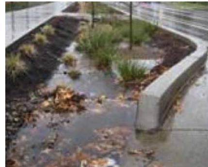
*Potential drywell solutions include constructing vegetated swales or rain gardens as shown here. These types of facilities collect stormwater and provide natural filtration as water returns more slowly to underground aquifers. Other potential solutions include constructing an underground piped system to connect to the existing municipal stormwater system.*
