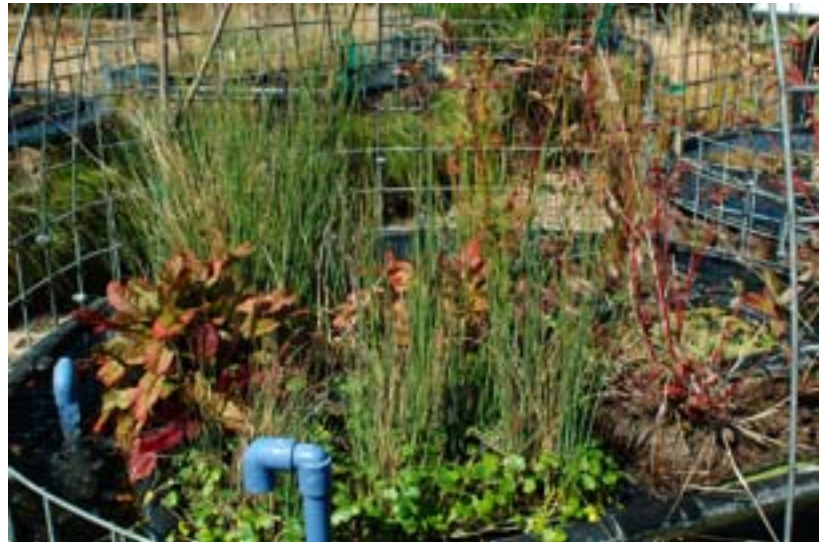
Above and to the left are small-scale plant treatment systems for graywater. The treatment tanks have 'living walls' - which are irrigated by the graywater. This system was built by Paul Kay for demonstration purposes at the Oregon Garden in Silverton.
