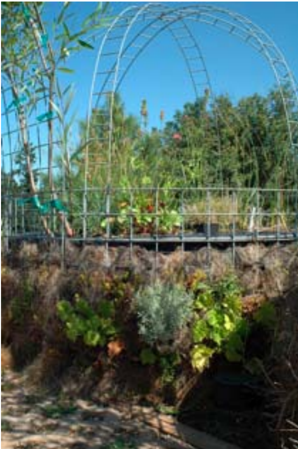
Above and to the left are small-scale plant treatment systems for graywater. The treatment tanks have 'living walls' - which are irrigated by the graywater. This system was built by Paul Kay for demonstration purposes at the Oregon Garden in Silverton.
