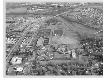
Eugene-Springfield Wastewater Treatment Plant Established 1984
