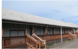
ShelterCare Homeless Recuperation New roof, stucco, paint, storage room
